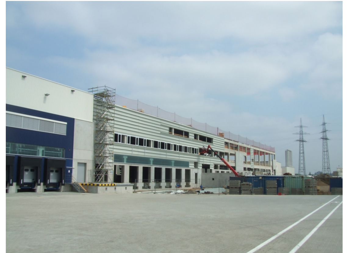
photo during the extension 4. CP
