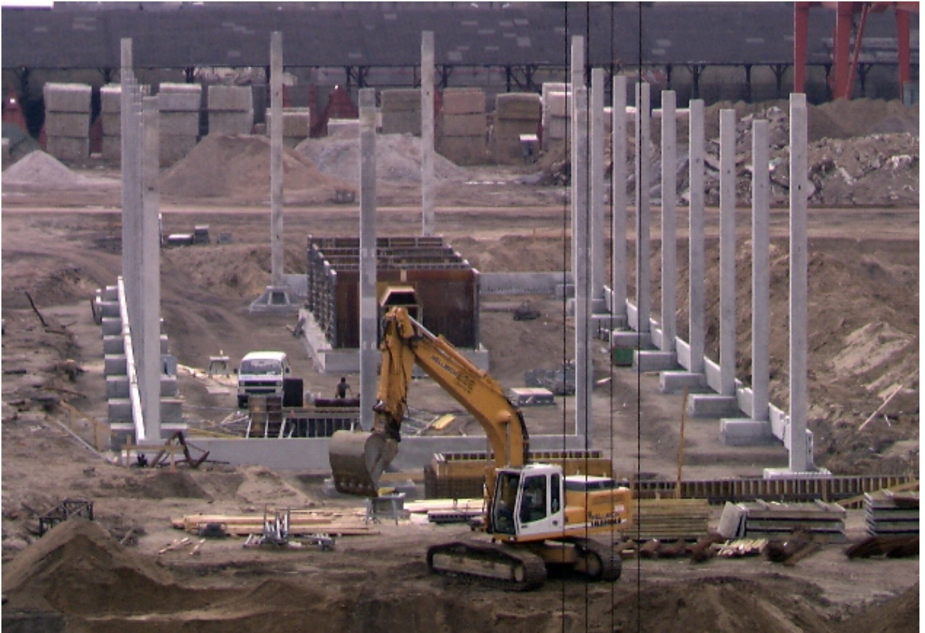
reinforced-concrete prefabricated steel stanchion of the debarker / chipper building (EZ), in the middle: formwork for the debarker drum
