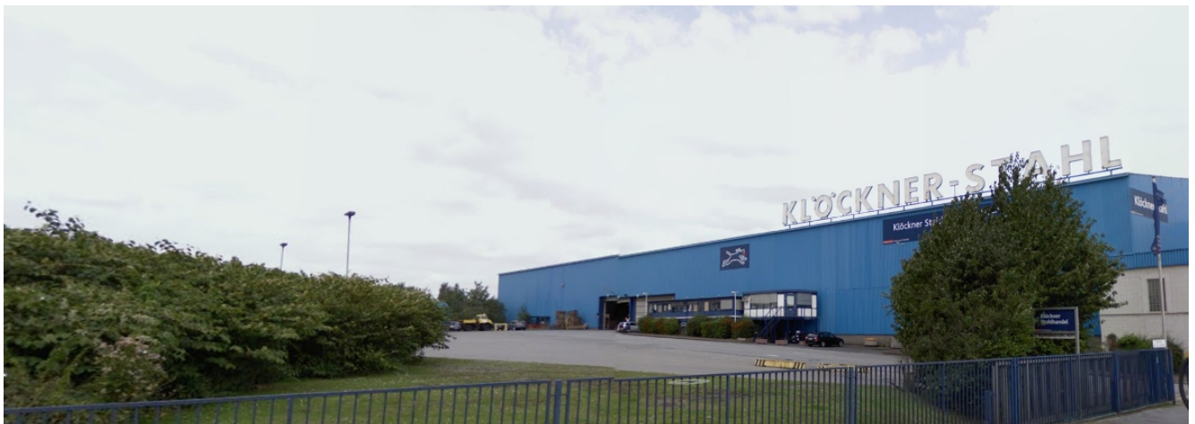
plant gateway (existing building stock)
