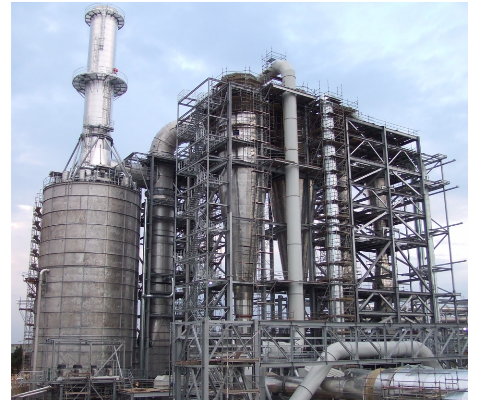
dryer framework during construction phase
