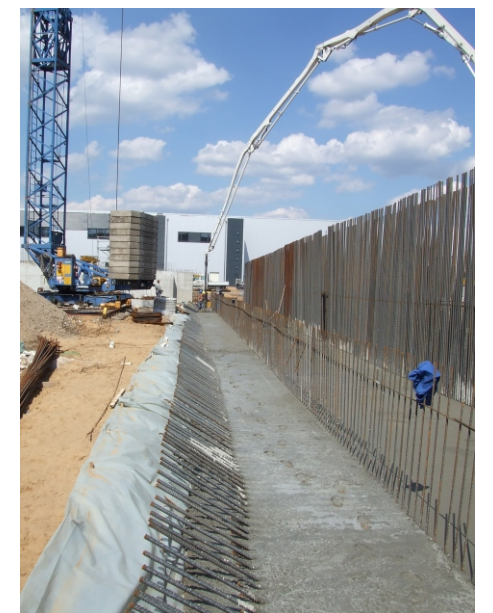
photos of the reinforcement work of the base plate discharge-canal
