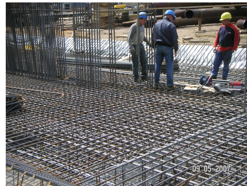
photos of the reinforcement work of the base plate discharge-canal
