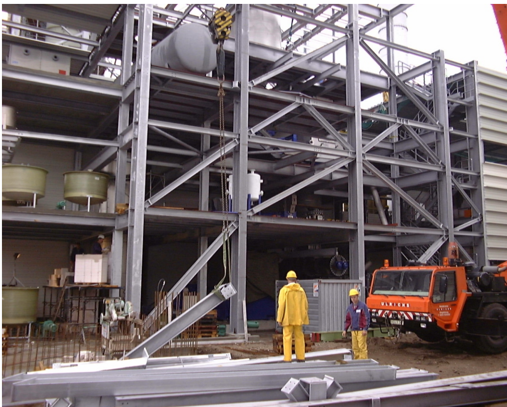
refiner / washer (RW) during construction
