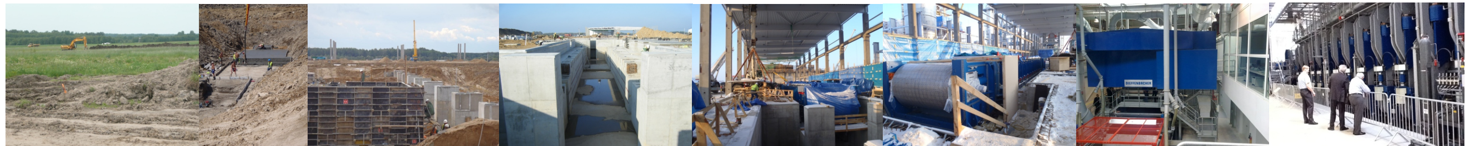
various construction stages press foundation
