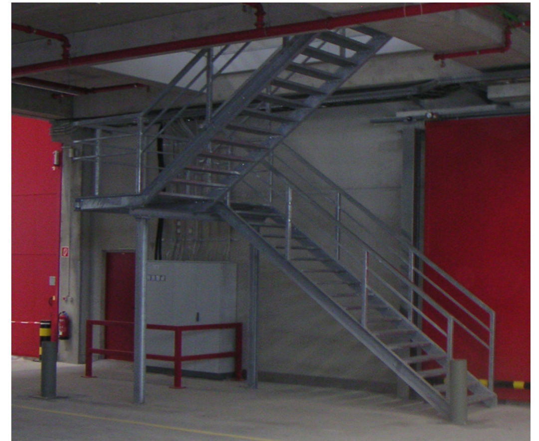
inside staircase warehouse office
