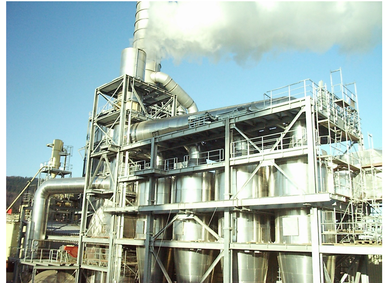
photo framework and combustion chamber, seperating cyclone and emergency stack over the drum dryer
