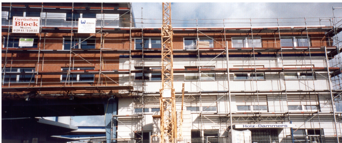
elevation during construction phase
