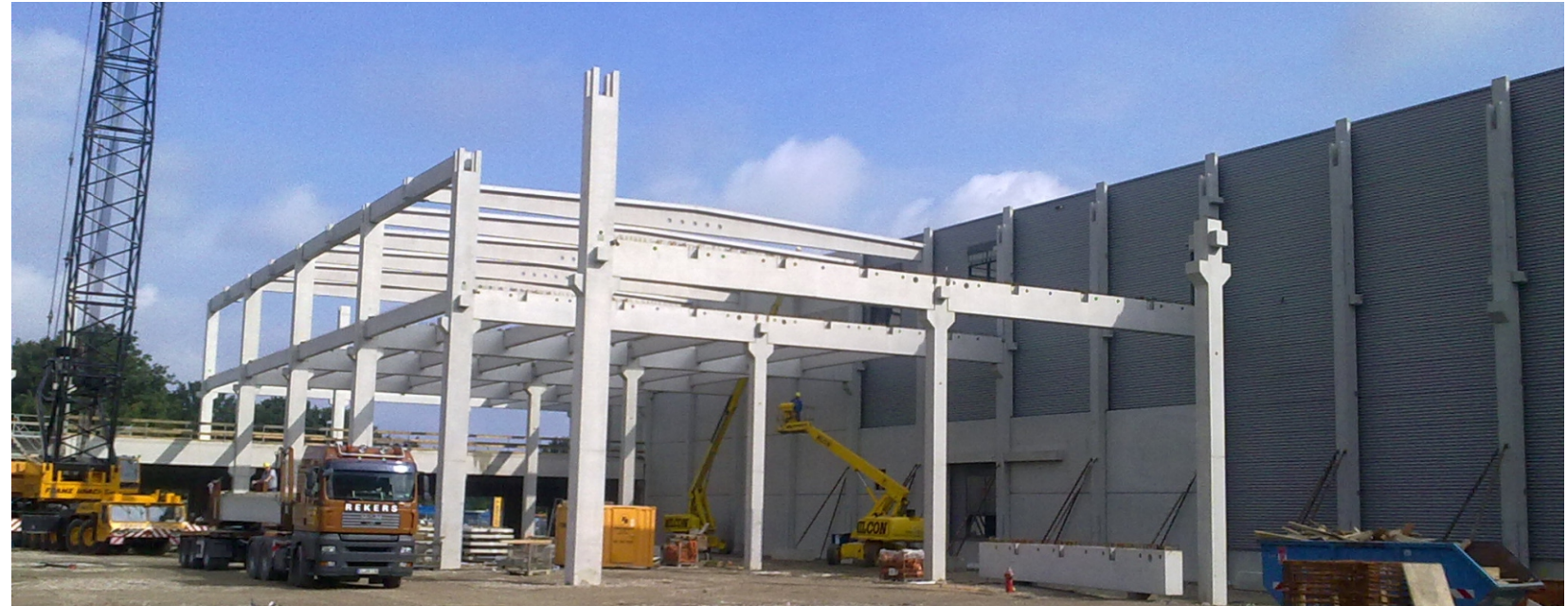
prefabricated construction hall A
